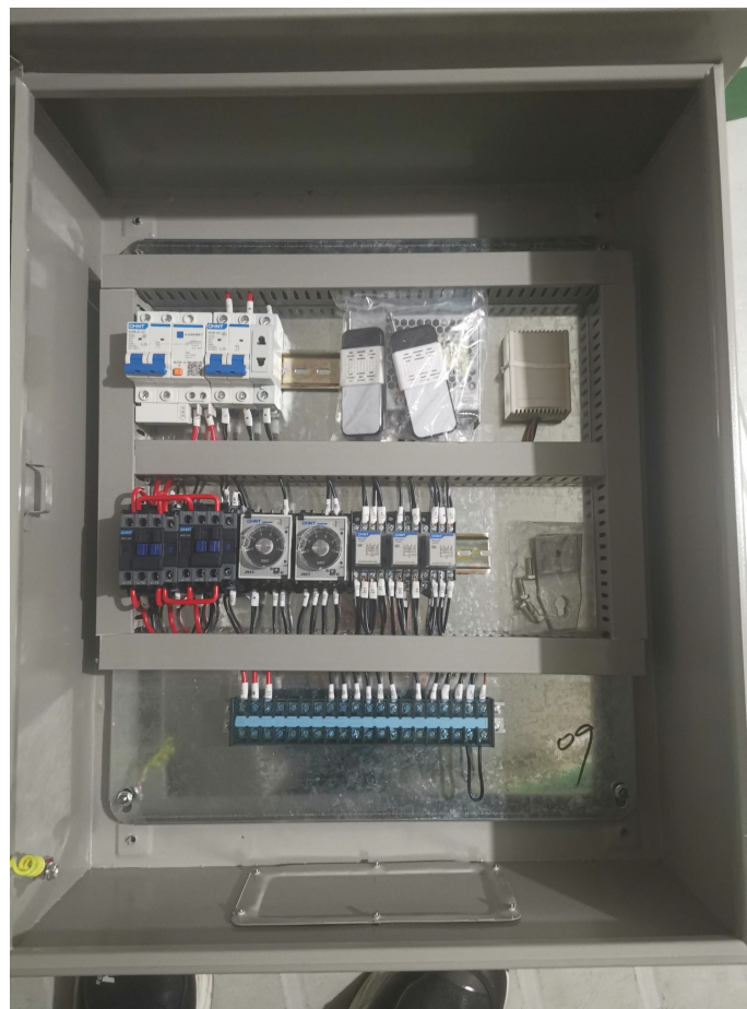
Internal layout diagram of the control system
